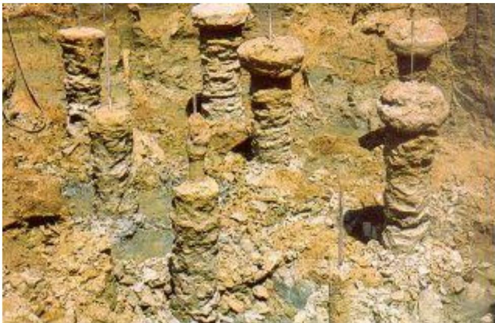
**Figura A.3-7: Aspecto final das colunas de *Jet-grouting*.**
