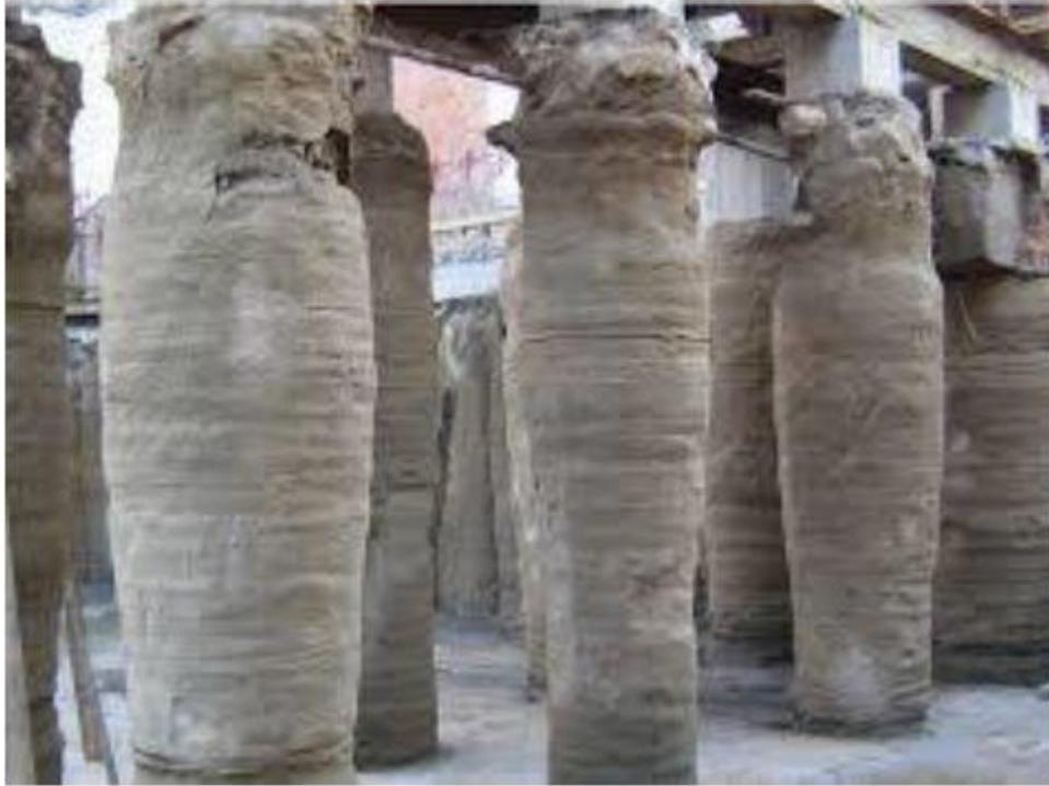
**Figura A.3-6: Aspecto final das colunas de *Jet-grouting*.**
