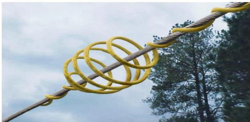
Figura 18 - Bird flight diverter BFD
