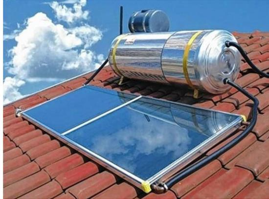
Figura 2. Colector solar plano
